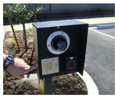
Photo: Pedestal-mounted card reader. Courtesy of United States Marshals Service (USMS).
